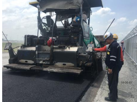
Pave asphalt concrete perimeter road (Airfield)
