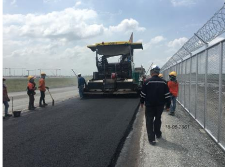
Pave asphalt concrete perimeter road (Airfield)
